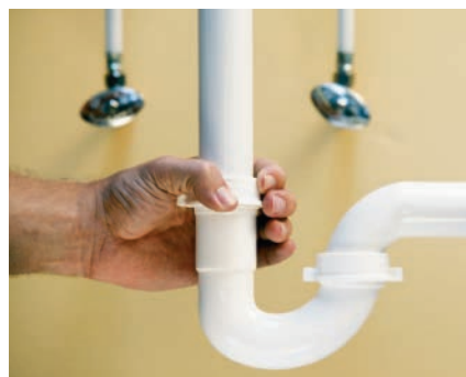
▲ FIGURE 12.24 Polyvinyl Chloride Polyvinyl chloride is used for many plastic plumbing supplies, such as pipes and connectors.
