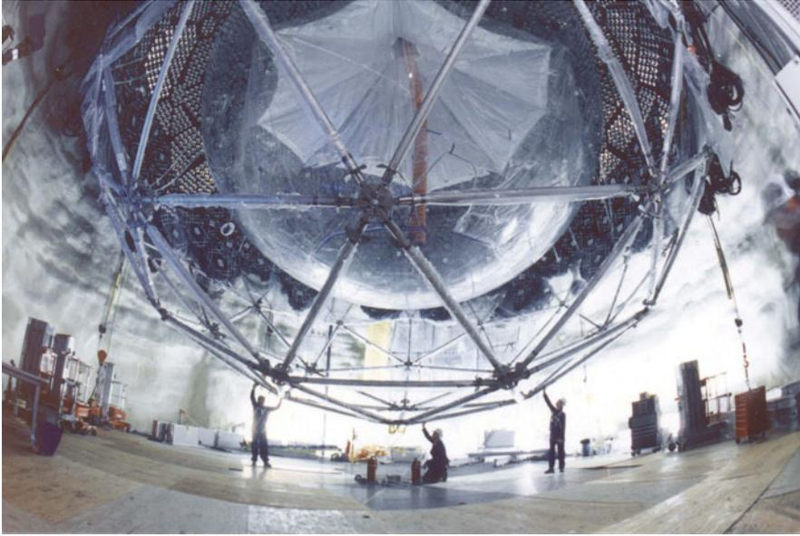
Plate 14.16 SNO detector during construction, showing the inner acrylic vessel and the outer cage partially populated at the top with photomultipliers. Courtesy of SNO.
