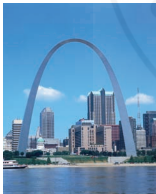
FIGURE 6 The St. Louis Arch has the shape of an inverted hyperbolic cosine.
