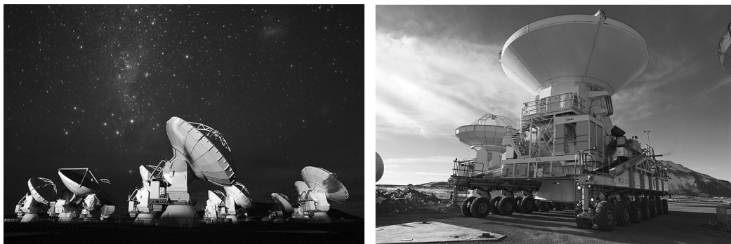
FIGURE 2.26 Left, Some of the individual radio telescopes making up ALMA. Seen at night. (Courtesy of Atacama Large Millimetre Array [ALMA]) (European Southern Observatory/National Astronomical Observatory of Japan/National Radio Astronomy Observatory [ESO/NAOJ/NRAO], C. Padilla.) Right, Moving one of ALMA's radio telescopes to a new site. (Courtesy of ALMA [ESO/NAOJ/NRAO], S. Rossi [ESO].)
